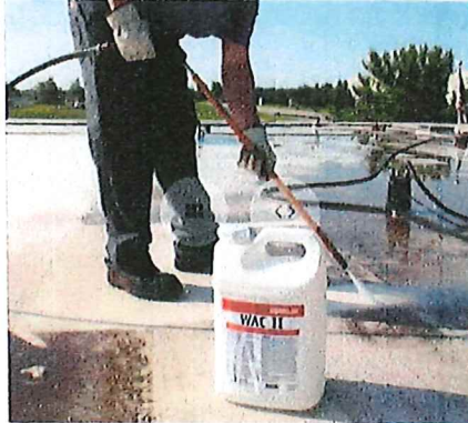
Wash with WAC cleaner and pressure washer
