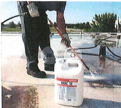
Wash with WAC cleaner and pressure washer
