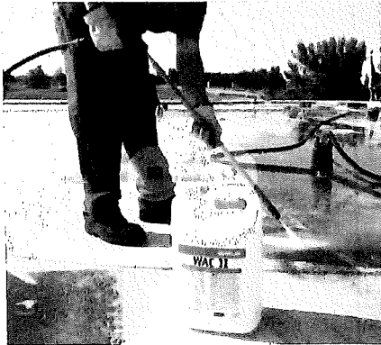
Wash with WAC cleaner and pressure washer
