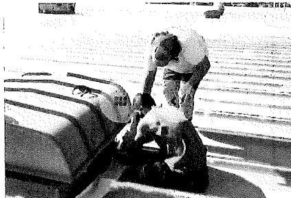
Apply Base coat and fabric around all skylights and protrusions
