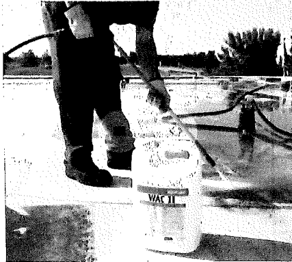
Wash with WAC cleaner and pressure washer
